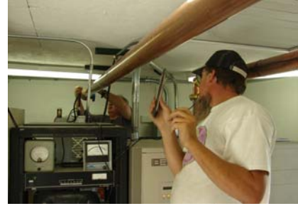
Mike and Sam 'plumbing' the transmitter
